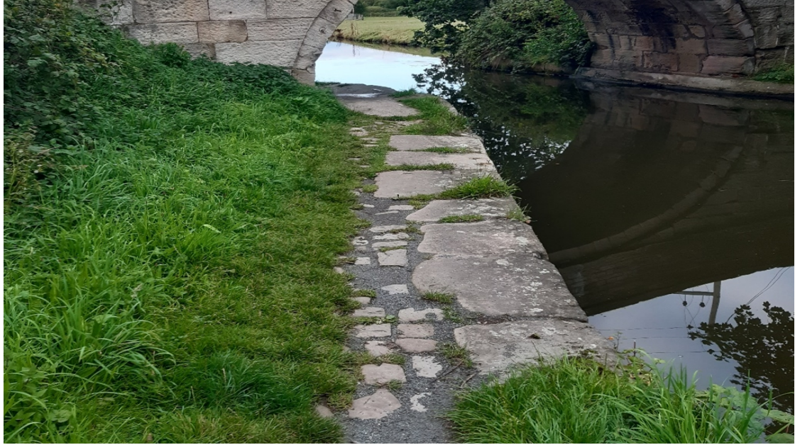
4 - North Moor Lane Bridge
